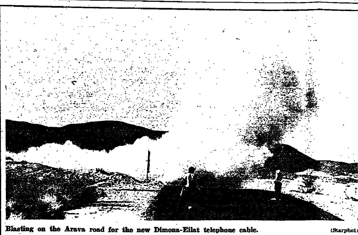
Blasting on the Arava road for the new Dimona-Eilat telephone cable. (Starphoto)
